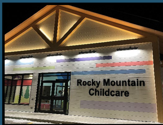
An Open House was recently held at Rocky Mountain Childcare, adjacent to Marysville Elementary School, to celebrate the completion of the new facility.
