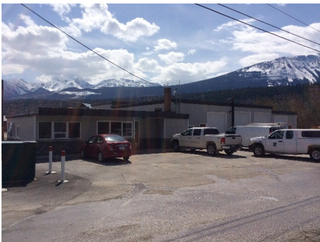
Signature - Exterior Elevation Golden Zone Office / Maintenance Building Auditor Touch Photo
